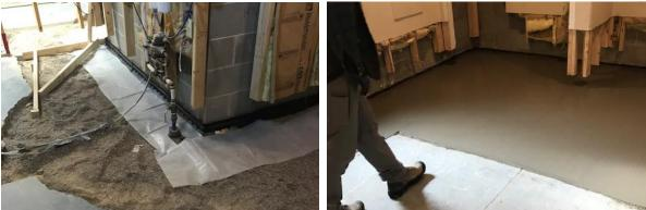
After the push piers and interior drain tile system were installed the concrete floor could be poured back into the basement, and once cured the rest of the remodeling could be completed. Now the homeowner may rest assured that the house is on a stable and dry foundation and will be for the life of the home. The project was completed in February of 2020.
